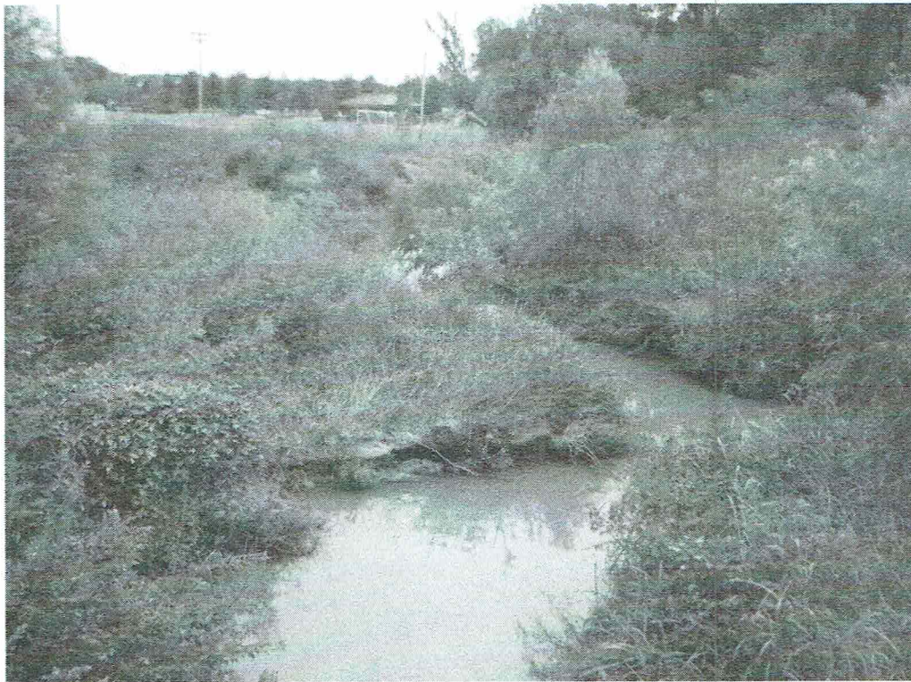
Looking downstream from culvert (August 23, 2012)
