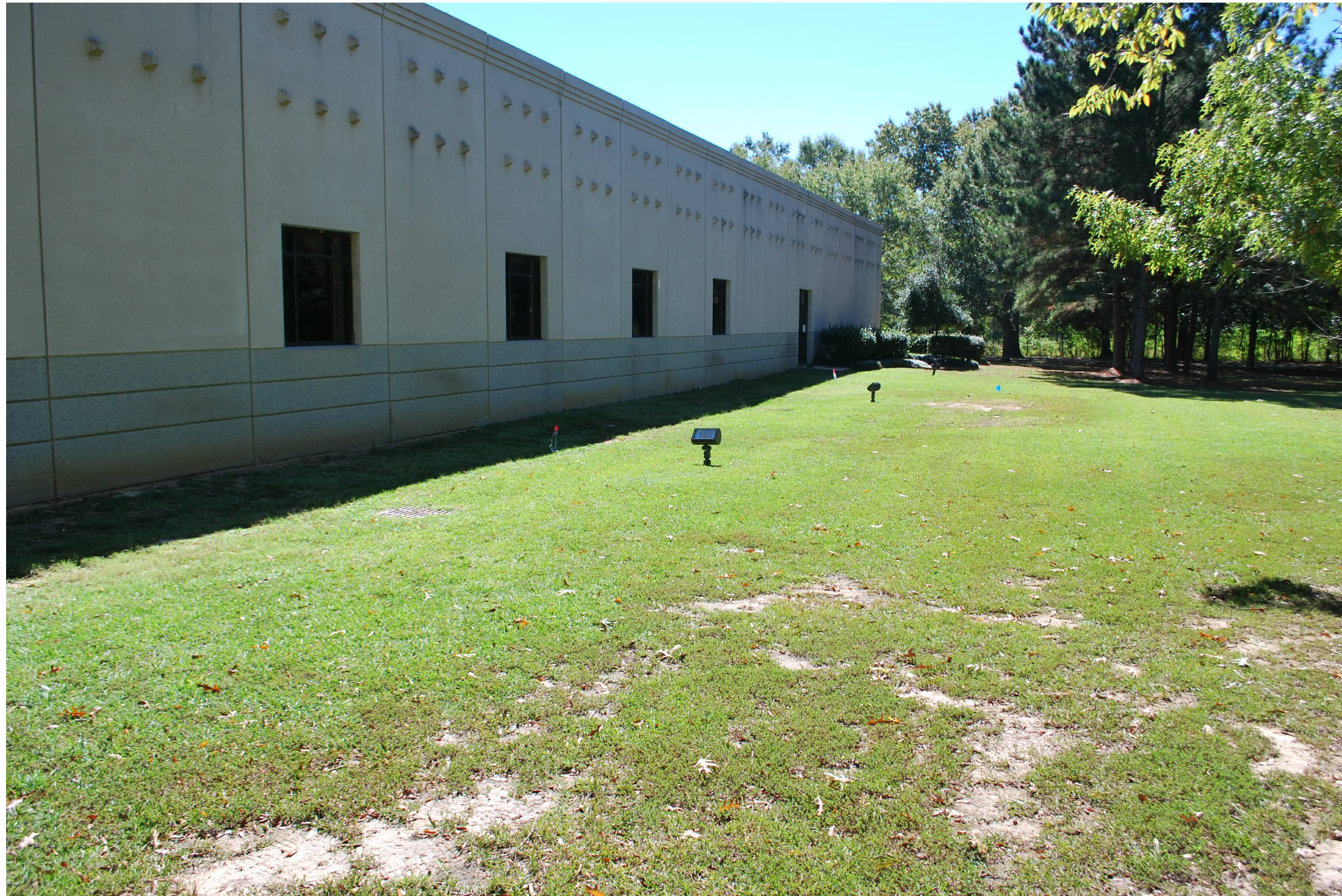
EXISTING PHOTOGRAPH OF WEST SIDE OF "ASSEMBLY" PORTION OF BUILDING - LOOKING SOUTH
