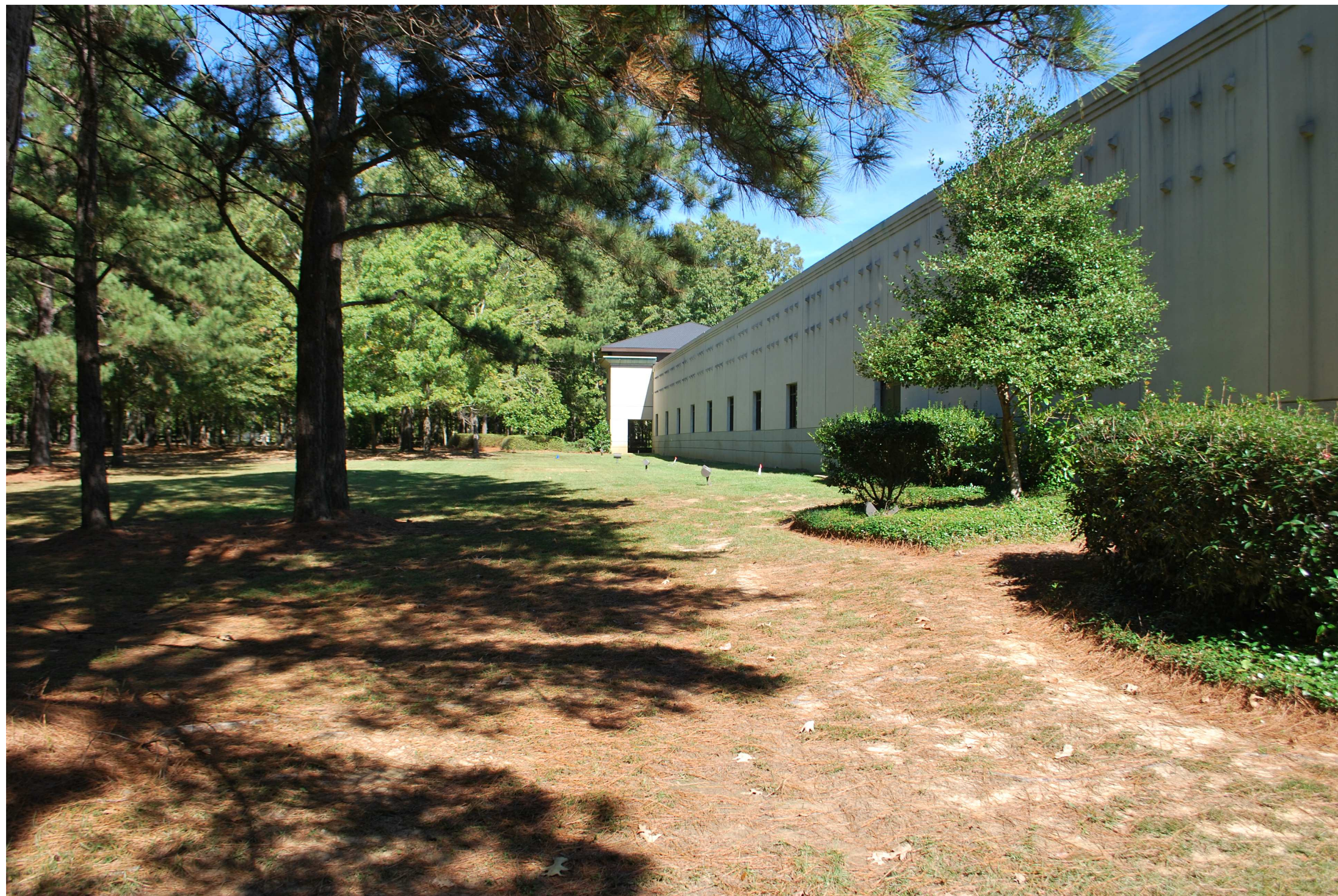
EXISTING PHOTOGRAPH OF WEST SIDE OF "ASSEMBLY" PORTION OF BUILDING - LOOKING NORTH
