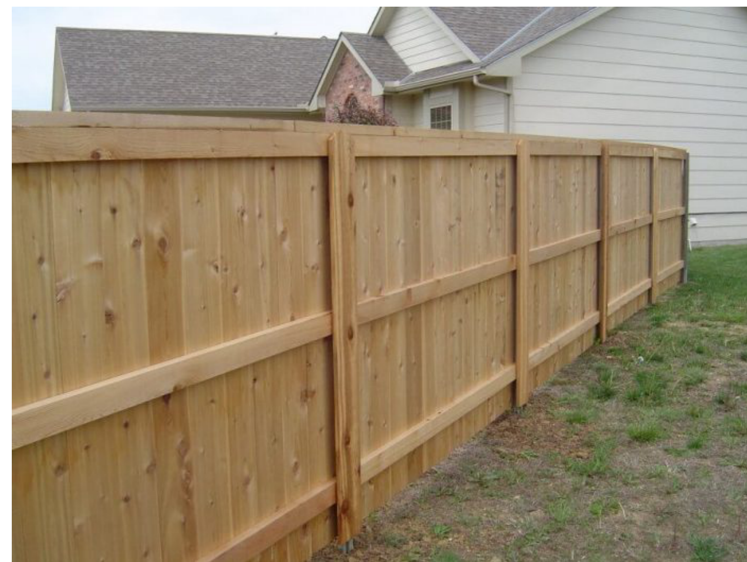
6' GOOD NEIGHBOR STYLE FENCING
