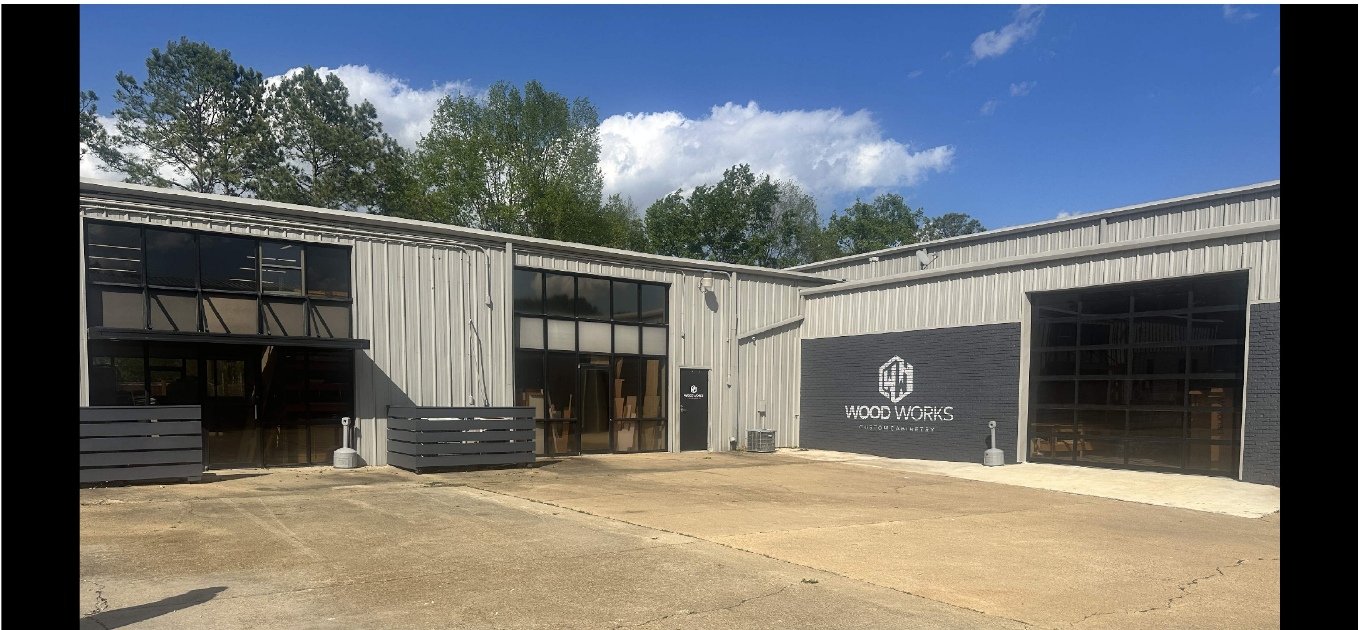
EXISTING SOUTH VIEW
