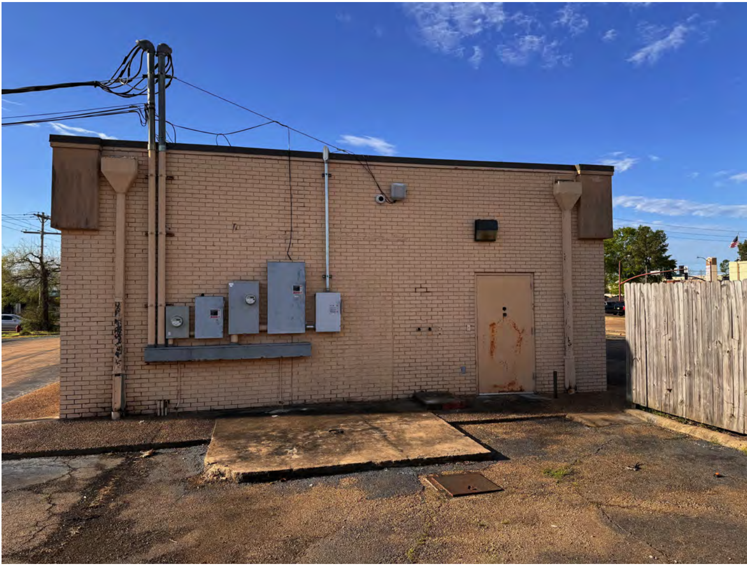
5 North (Back of building) A202
