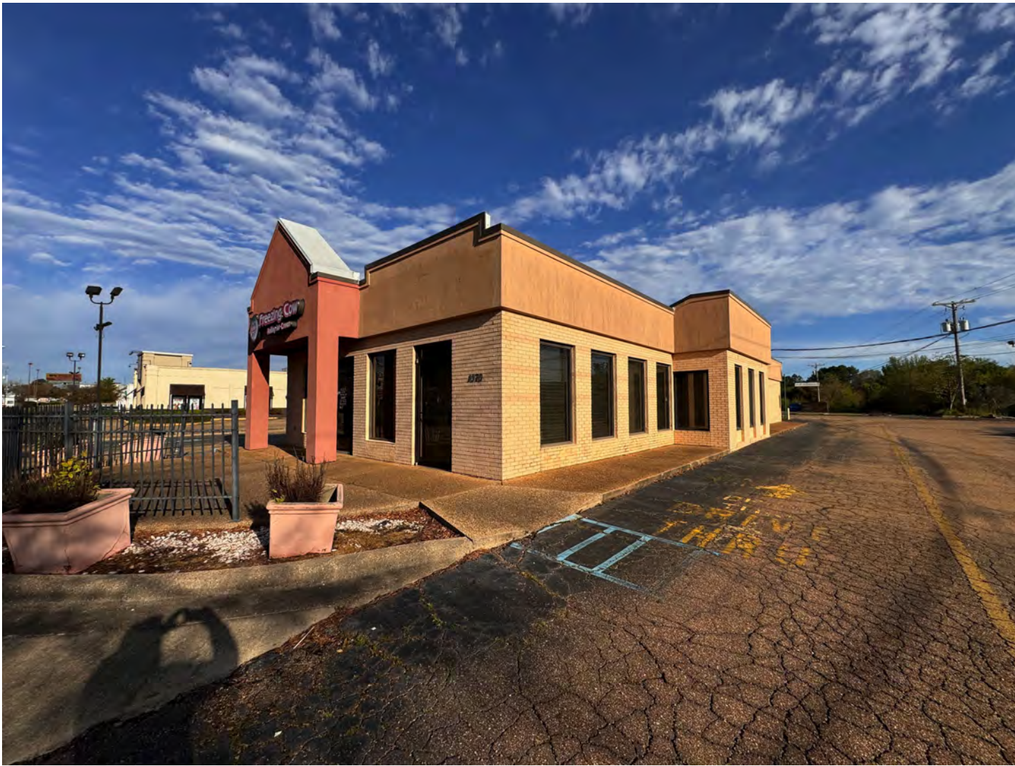
2 Southeast Corner A202
