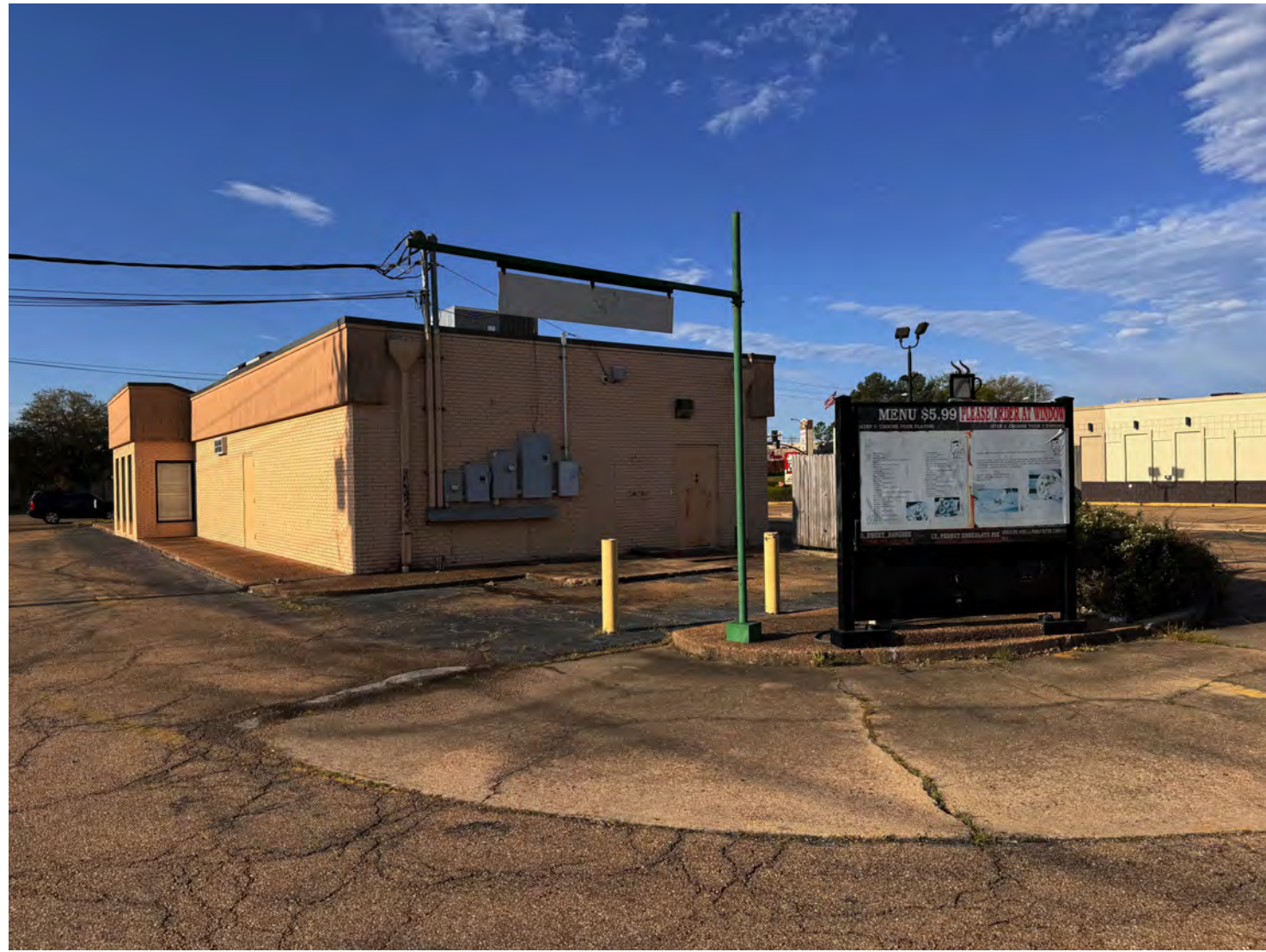
4 North (Back of building) A202
