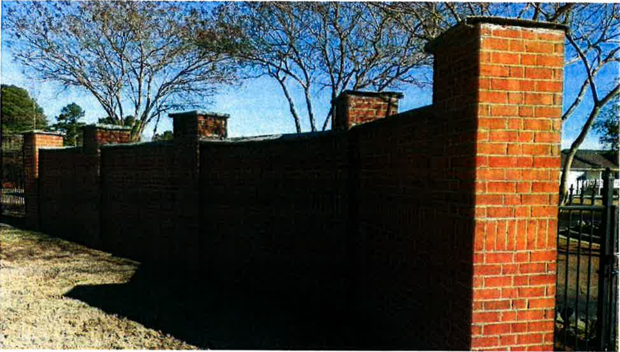
Entrance Sign Caps:
