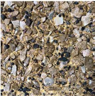
CONCRETE WALL PANEL - EXPOSED AGGREGATE
