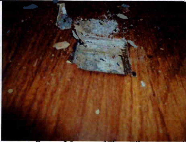
Core – 8 Layers of Floor Tile
