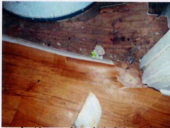
1 st and 2 nd Layers of Wood Vinyl Sheet Flooring
