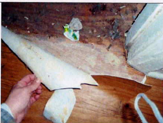
Yellow Mastic associated with 1 st Layer of Flooring
